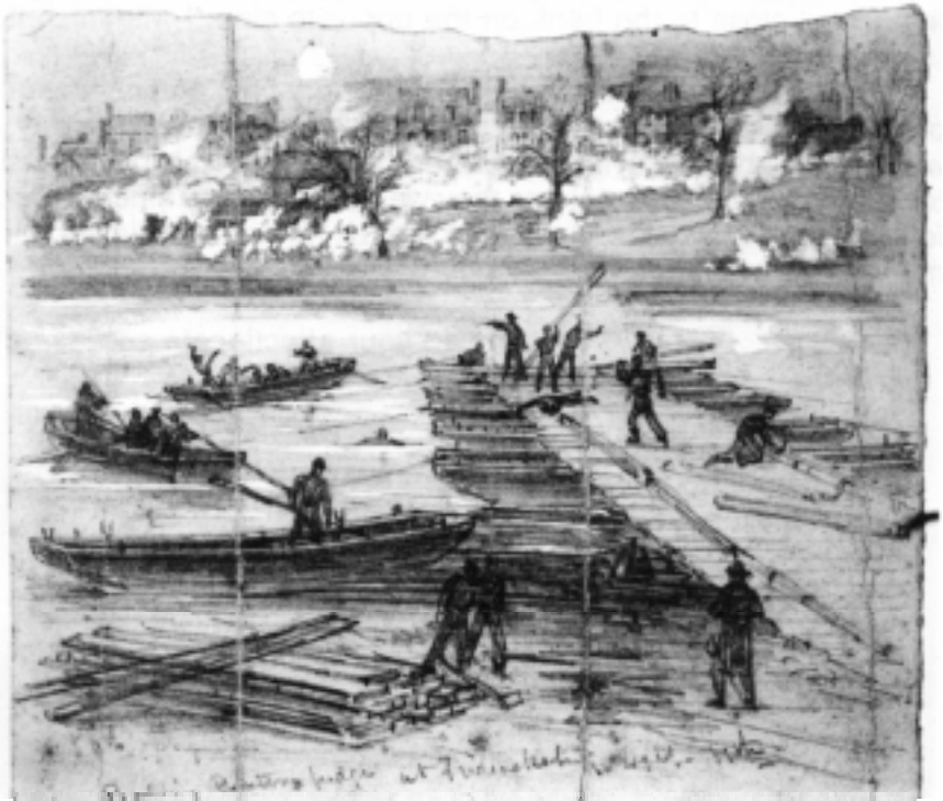
Sketch of Engineer troops laying ponton bridge at Fredericksburg, Virginia, 11 December 1862, by Alfred R. Waud. Library of Congress photograph Z62- 7023.
